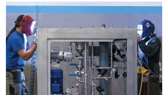
Orbital welding of pipes
